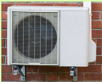
**Heat pumps** are extremely efficient, using one unit of electrical energy to bring about three units of heat into your home.
